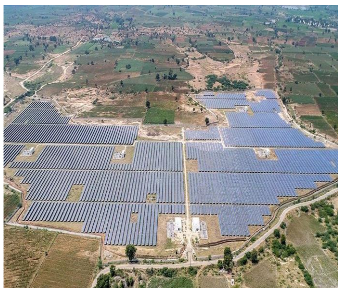
Megawatt scale solar system
